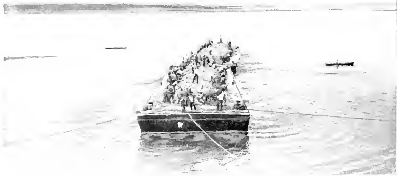
MAT SINKING: THE FINISH.
